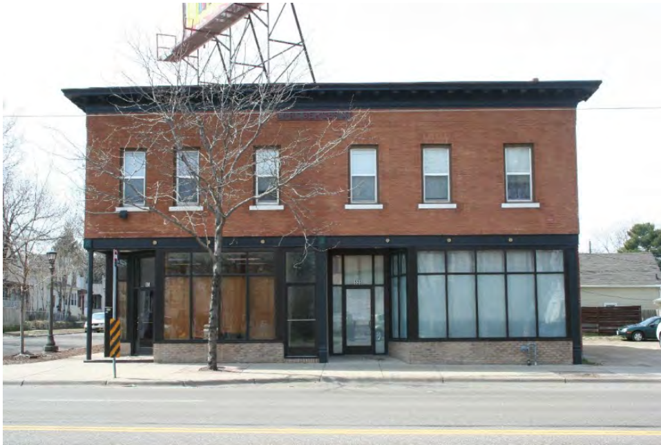
The R.C. Berger Building, located at 535 Dale Street, is an intact example of early twentieth century commercial development along Dale Street. View facing west.
