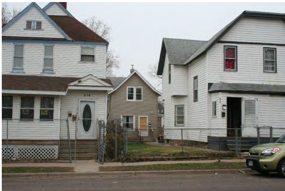
Example of an alley house, located between 514 and 516 Thomas Avenue. View facing south.
