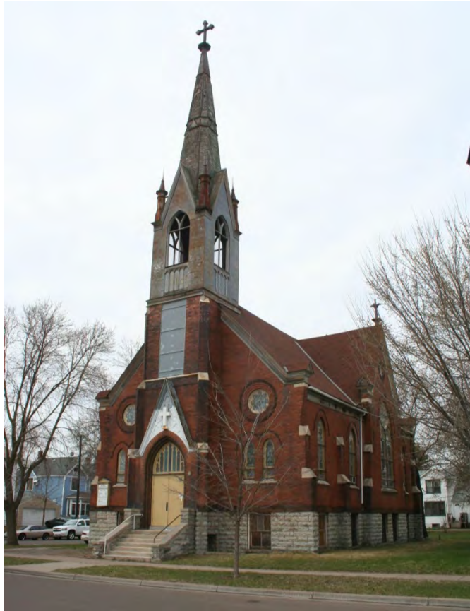
The Norwegian Evangelical Lutheran Church (1870) at 515 Farrington Street stands as an intact example of early ecclesiastical architecture in the survey area. View facing southwest.
