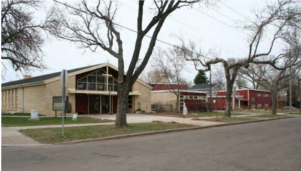
St. Peter Claver Catholic Church located at 375 Oxford Street North is an example of modest mid-century ecclesiastical architecture in the southwestern corner of the survey area. View facing northwest.
