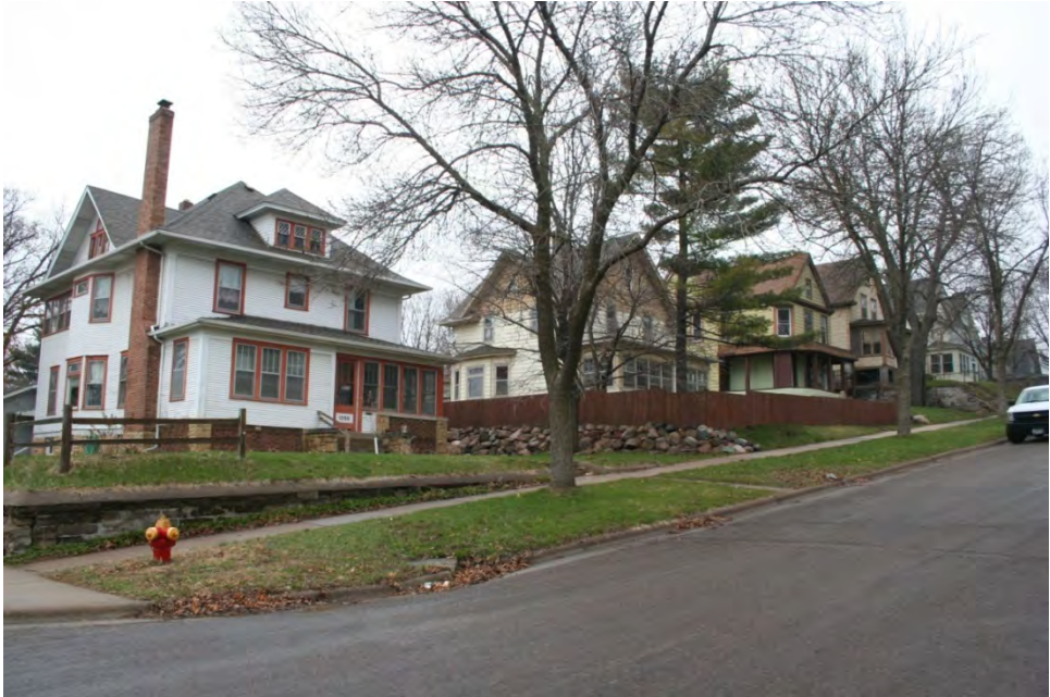
West side of Bradley Street north of Cook Avenue. View facing northwest.
