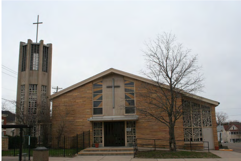
The New Hope Baptist Church at 712 Burr Street is an example of modern ecclesiastical architecture in the Payne-Phalen survey area. View facing east.
