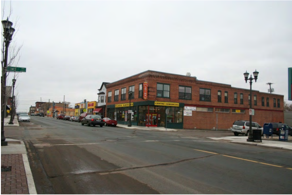
East side of Payne Avenue at Sims Avenue. View facing northeast.
