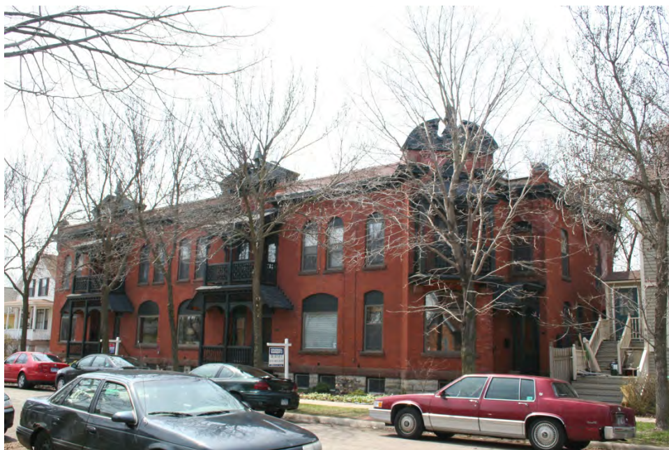
The Gardner Row House at 89 Leech is an example of a row house found in the West 7 th Street survey area. View facing southwest.
