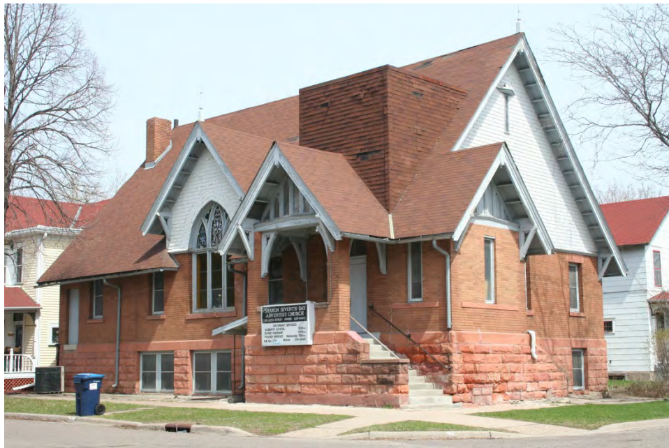
Central Church of Christ at 80 Leech Street, constructed in 1903, is the earliest extant church in the survey area. View facing northeast.
