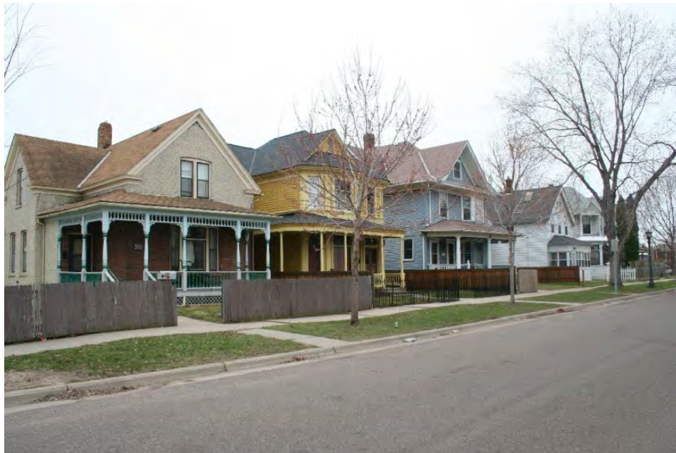
South side of Sherburne Avenue, mid-block, between Kent and Dale Streets. View facing southwest.
