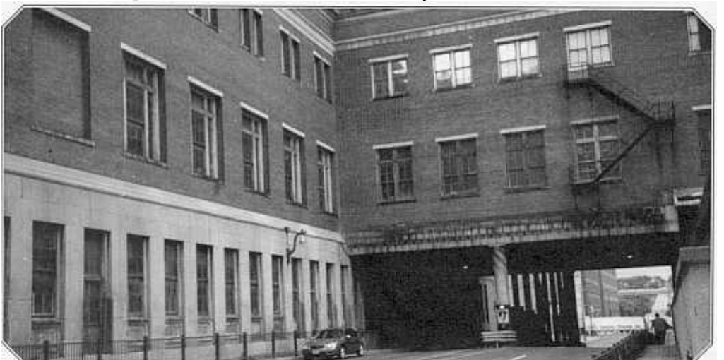
The back of Union Depot, along Kellogg Boulevard. This part of the building is in worse condition than the front lobby area.
